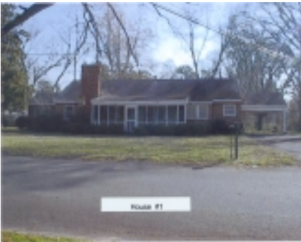
Milledgeville site targeted for renovation
